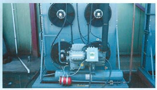
Blast chiller operating on RS-50 (R442A) which shows an increased energy efficiency of 22% and a higher capacity of 14% compared to R404A.
