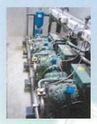
The system was originally designed for the refrigerant R-507 and in the end the only modification made for using R-442A (RS-50) was to slightly close the expansion valves due to its molecular structure being smaller than that of R-404A/R-507.
