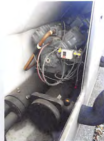
Semi-hermetic compressor with heat exchangers
